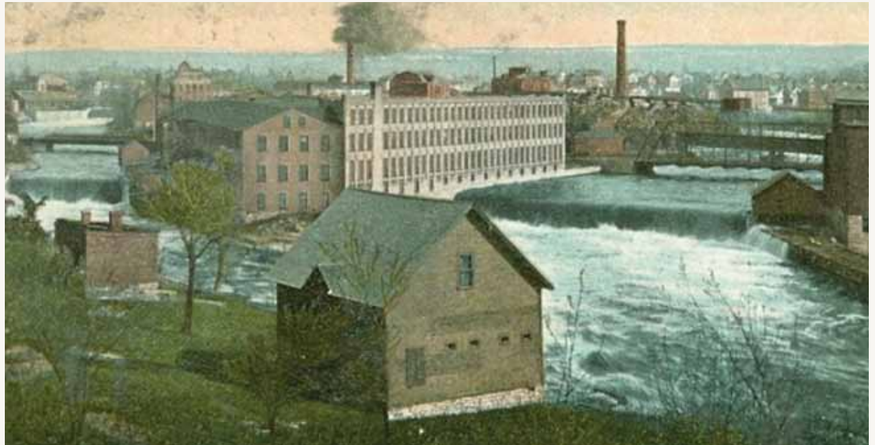
Watertown's industrial center along the Black River.
